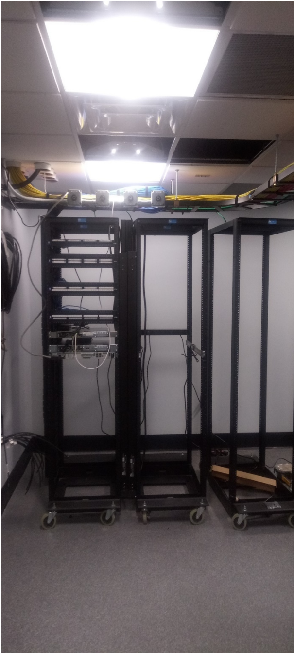
Server Room 122 – Pulling data wiring thru the F1 data rack continues.
