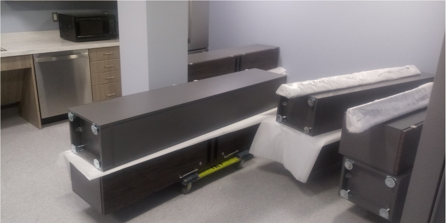
Xybix Locker delivery & installation.
