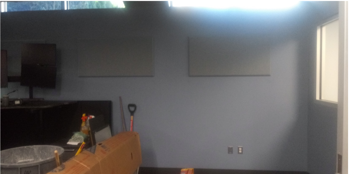
Dispatch 120 – Acoustical panel installations have been completed.
