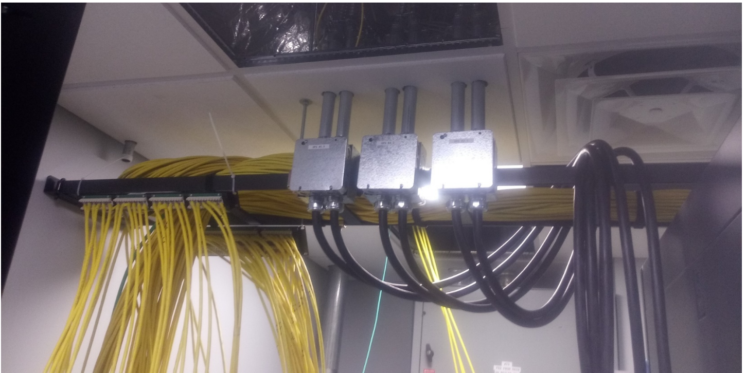
Server Room 122 – Pulling data wiring at cable tray continues.
