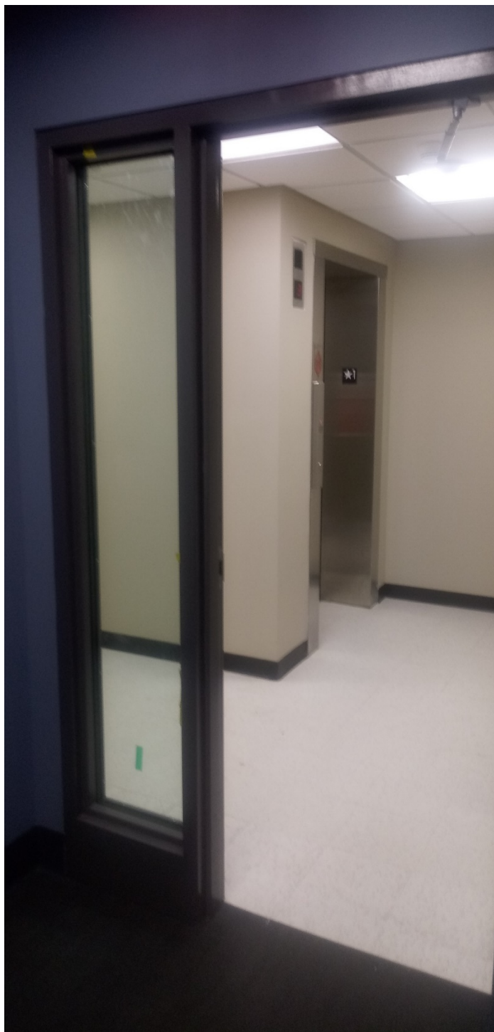
Opening 016 – Bullet resistant glazing has been installed.
