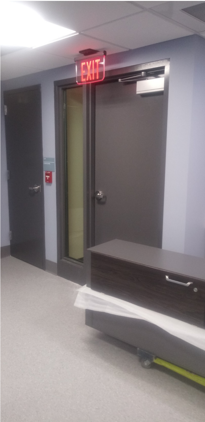
Opening 018 – Bullet resistant glazing has been installed.
